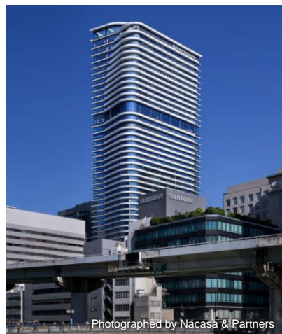
▲ Brillia Tower Dojima (Japan's first ultra-high-rise private residence housed in the Four Seasons Hotel)
