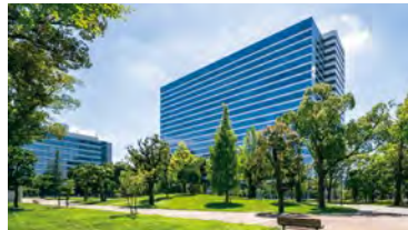
NAKANO CENTRAL PARK enables an efficient office layout through the use of a mega plate (for an uninterrupted single floor) measuring 1,500 tsubo (nearly 5,000 m 2 ) while offering a new style of working in an open, green environment. (Built in 2012).
