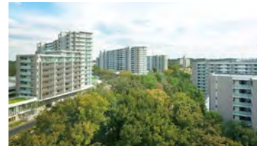
Brillia Tama New Town is Japan's largest apartment complex reconstruction project. (Built in 2013)
