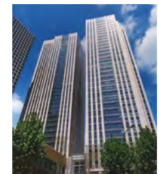
KASUMIGASEKI COMMON GATE is a pioneering public-private, large-scale redevelopment project executed using a private finance initiative (PFI) structure. (Built in 2007)
