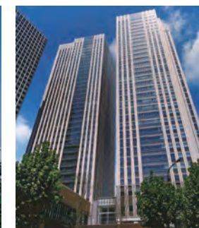
KASUMIGASEKI COMMON GATE is a pioneering public-private, large-scale redevelopment project executed using a private finance initiative (PFI) structure. (Built in 2007)
