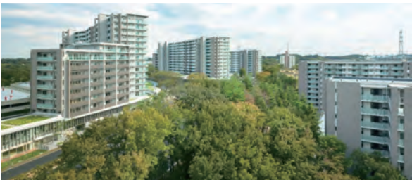
Brillia Tama New Town is Japan's largest apartment complex reconstruction project. (Built in 2013)
