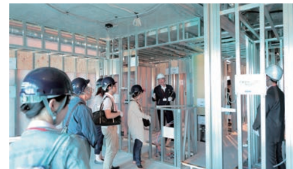
A construction site tour
