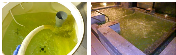
Water with hydrogen peroxide is cycled to sterilize pipes
