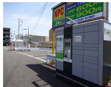
NPC24H Minami-osawa Station Front Parking (Outdoor Installation)
