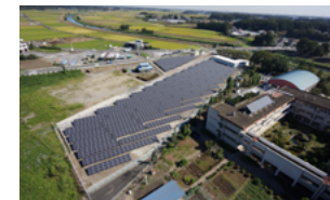
Oyama Solar Power Plant
