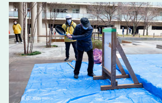
Training on breaking partition walls
