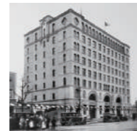
Exterior of Tokyo Tatemono Building
