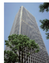
Shinjuku Center Building
