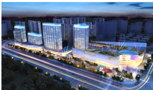
Xuzhou Qiaohu Project (Xuzhou City, China)
