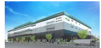
Logistics facility T-LOGI Kuki
