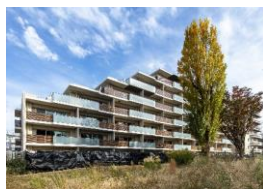
Brillia Oyama Park Front Integrated development: condominiums + childcare facilities
