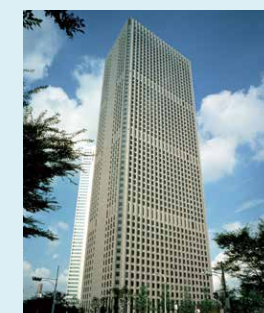
Shinjuku Center Building
