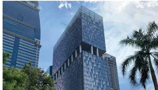
79 Robinson Road (CPF Building Redevelopment Project)
