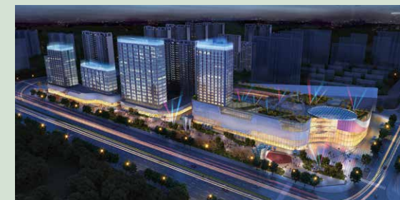
Xuzhou Qiaohu Project (Xuzhou City, China)
