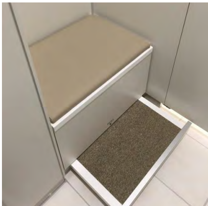
Installation of Bench with Fitting Board in Dressing Rooms
