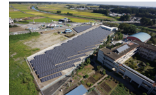
Oyama Solar Power Plant
