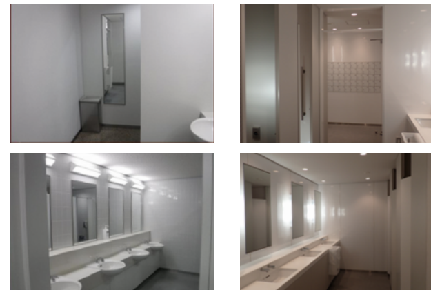
Shijo-Karasuma FT Square, restroom renovation work Left: Before renovation Right: After renovation
