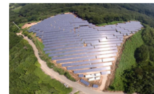
Hatoyama Solar Power Plant
