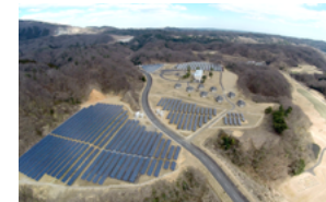
Iwaki Solar Power Plant
